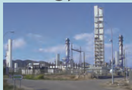
Energyworks Cartagena, Iberdrola, Spain
